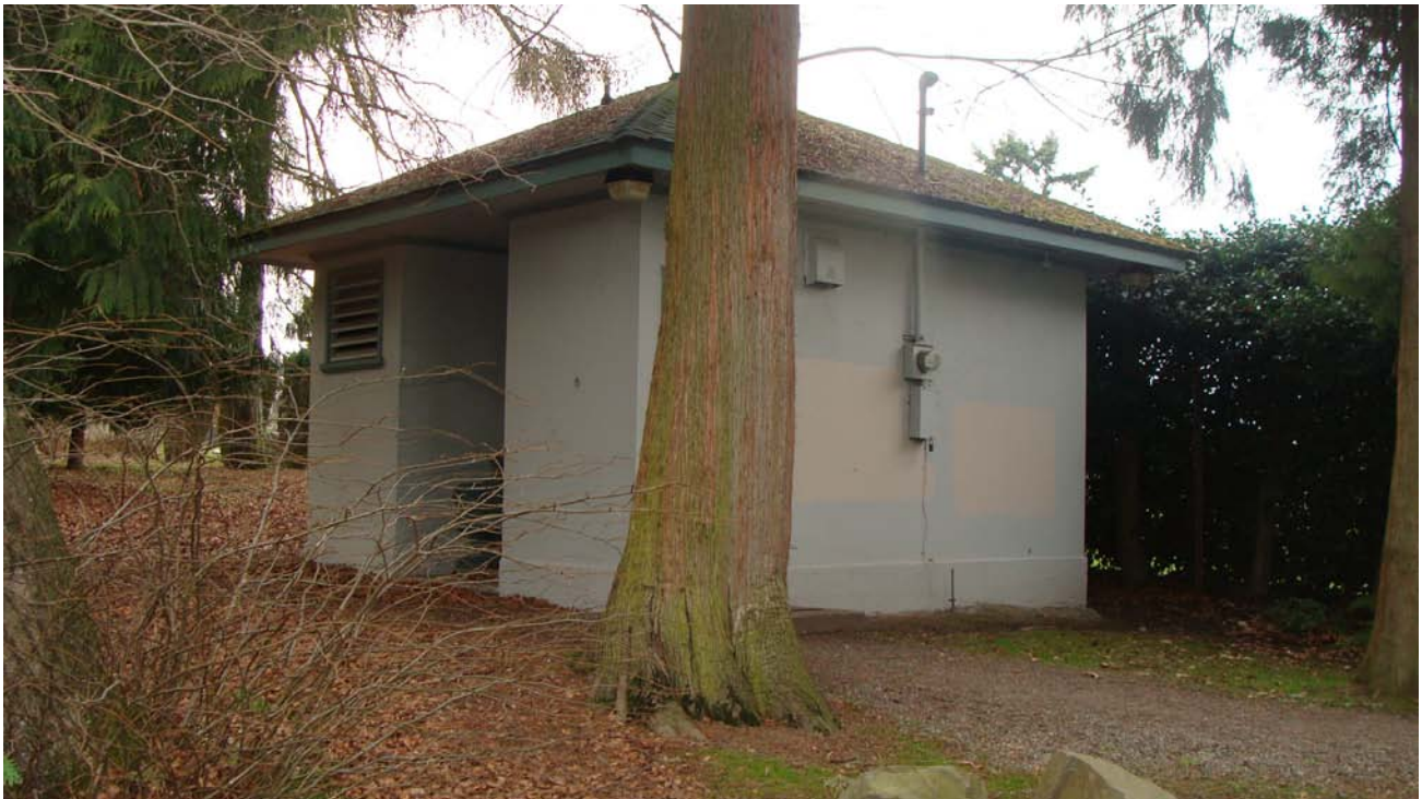
Photo 20 – Comfort Station, south and east sides, February 2009
