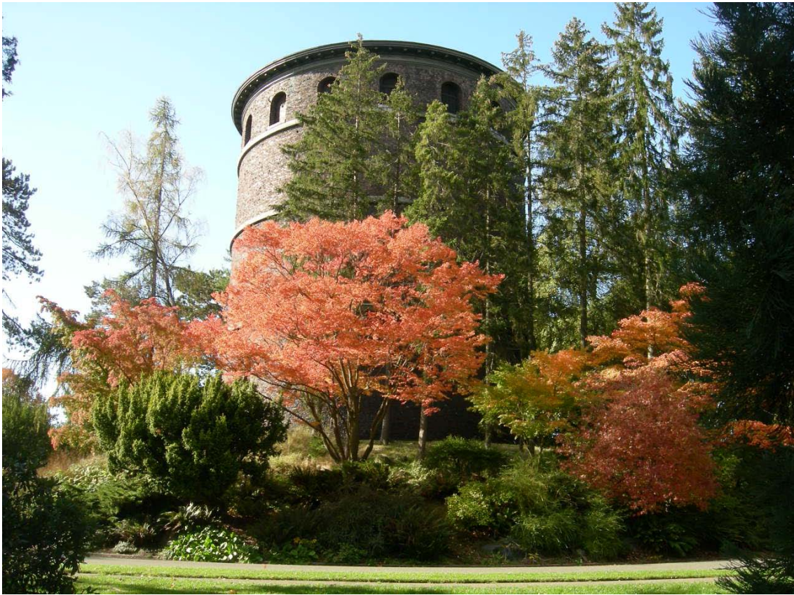
Photo 13 – Water Tower, east side, October 2010
