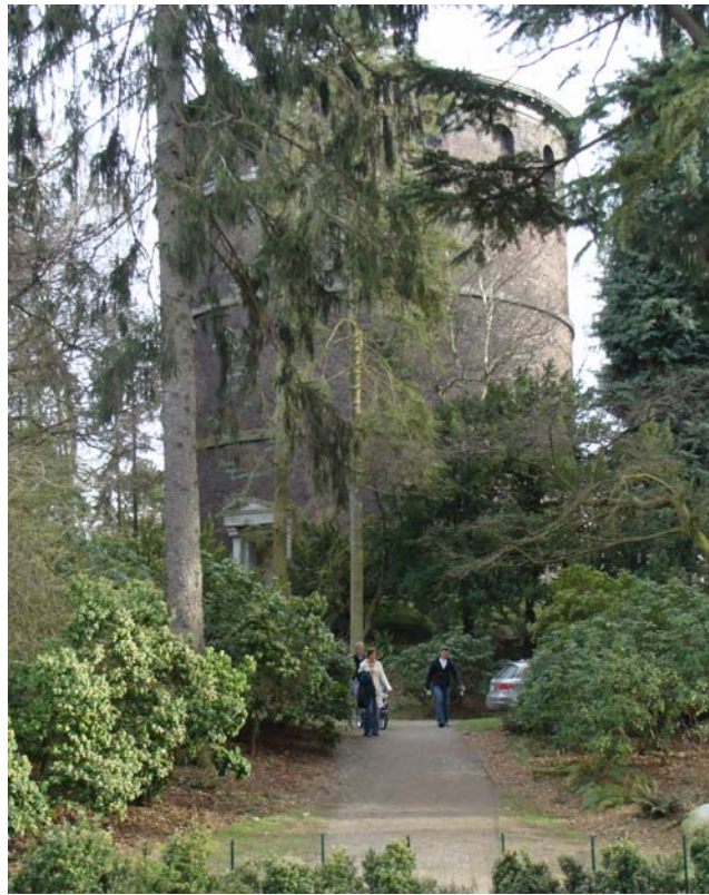
Photo 12 – Water Tower, northwest side, February 2009
