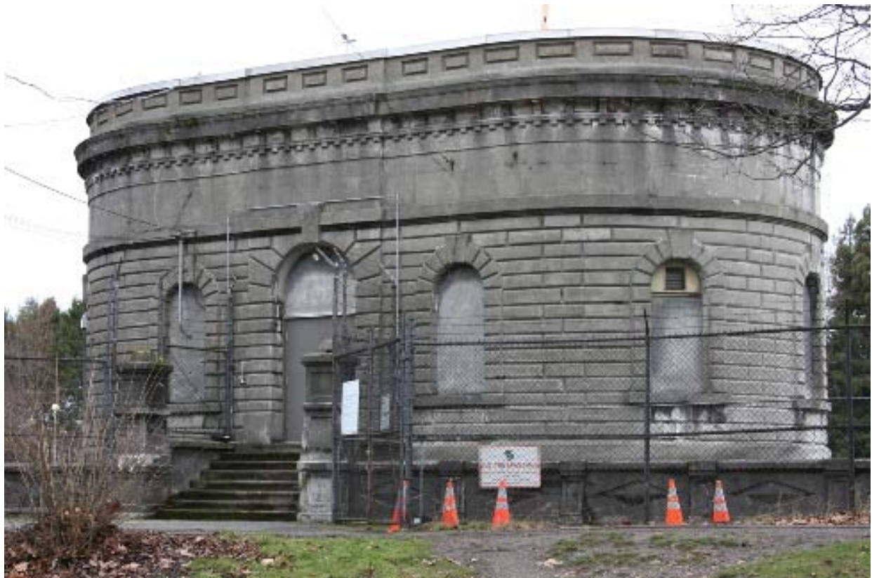
Photo 8 – Gate House, southeast corner, January 2007
