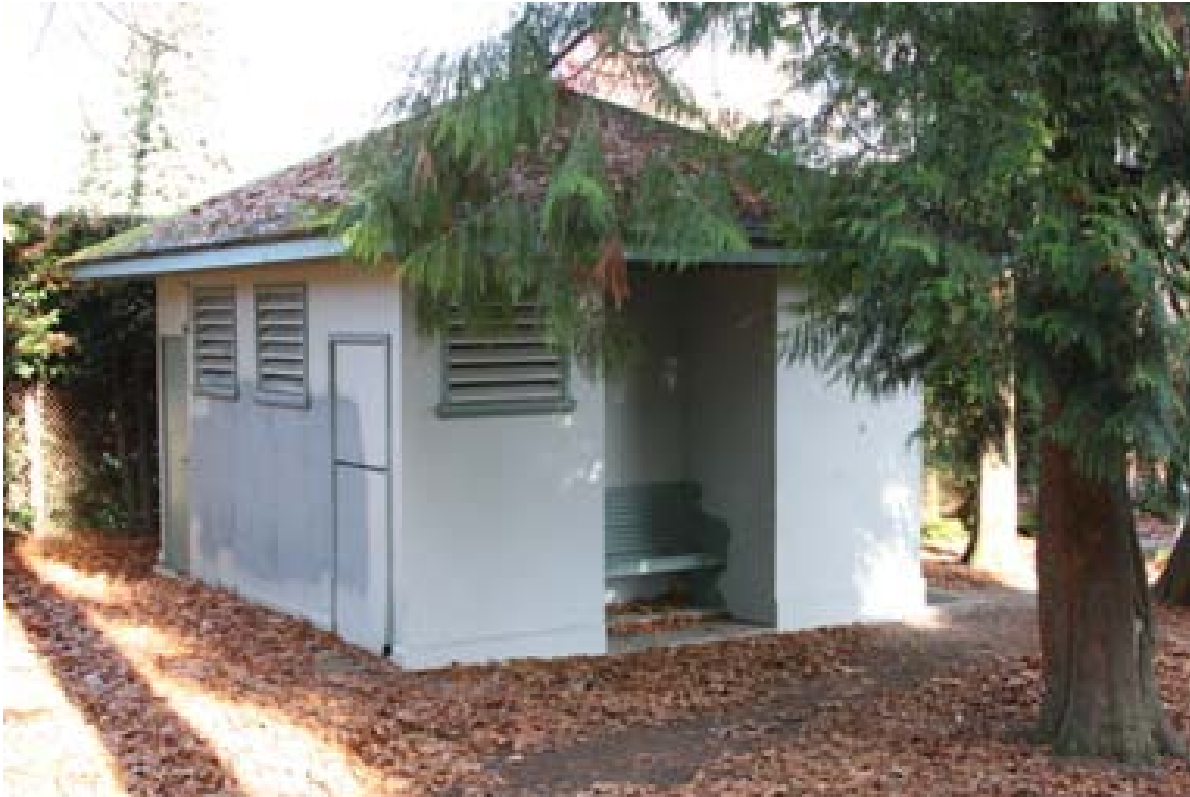
Photo 19 – Comfort Station, south and west sides, February 2008
