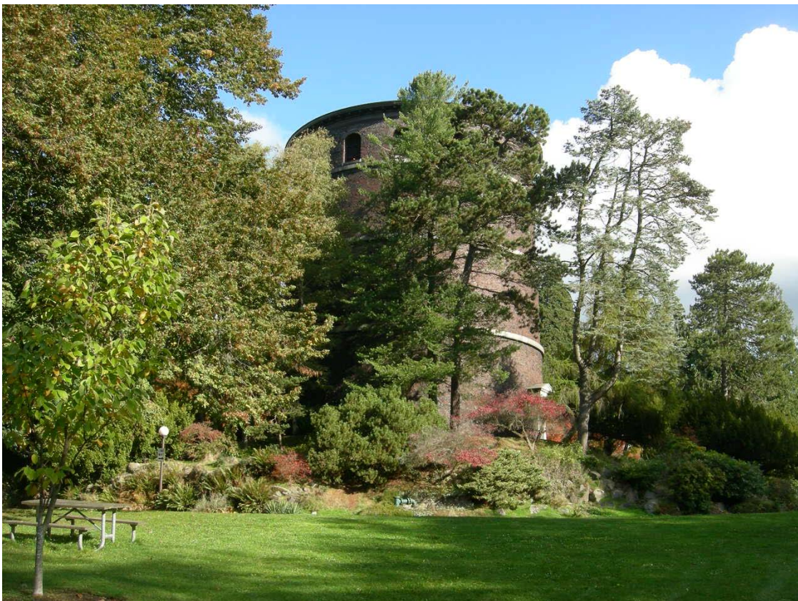
Photo 14 – Water Tower, west side, October 2010
