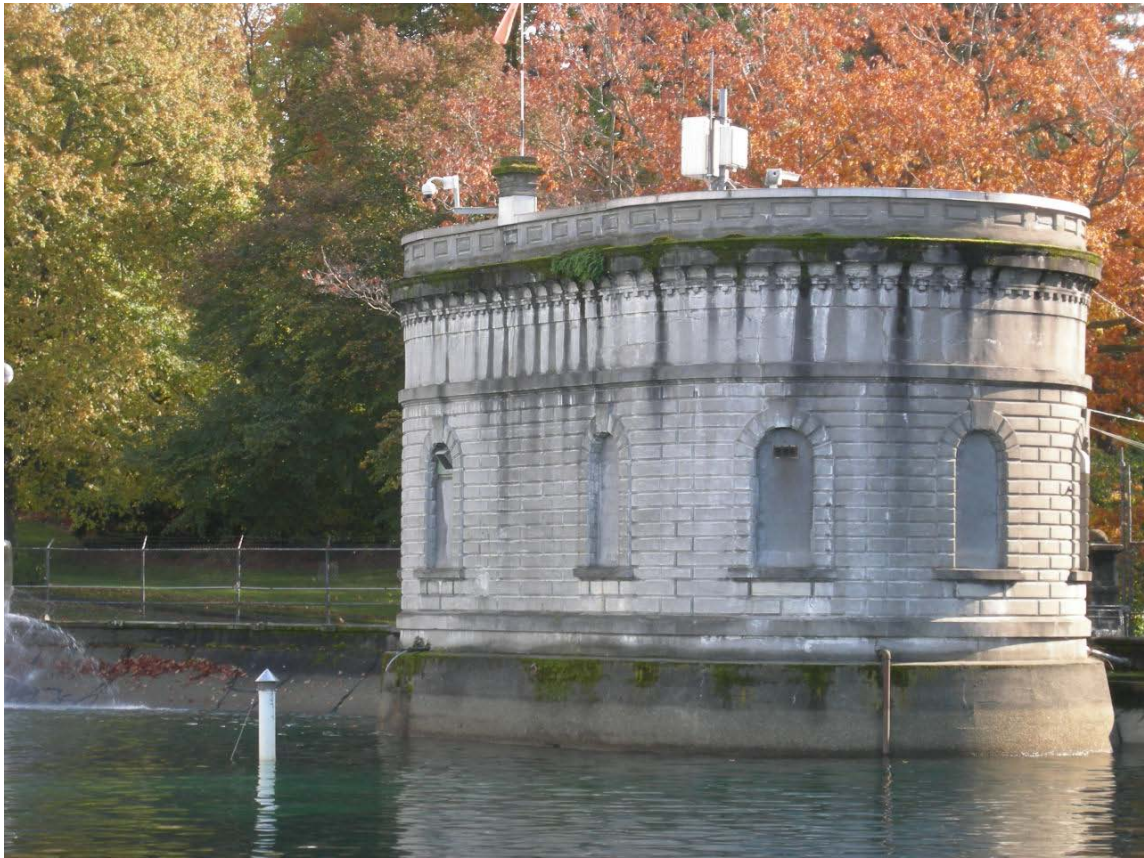
Photo 9 – Gate House, north side, October 2010
